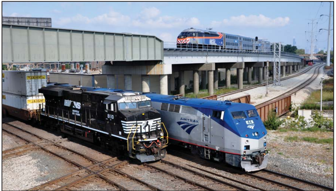
The new Englewood flyover bridge carries Rock Island trains over Norfolk Southern tracks used by freight and Amtrak trains.
